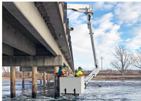
In cooperation with the Idaho Transportation Department, we are installing sonar depth sensors on three bridges to provide real-time monitoring for bridge scour. The three sensors will be connected with existing streamgauge stations on the [Boise River near Parma](#) in Canyon County, the [Payette River near Letha](#) in Gem County, and the [St. Joe River at Calder](#) in Shoshone County.
